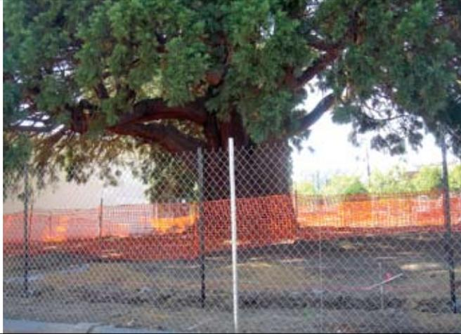
**Ideal Fencing Materials:** Trees to be preserved may be protected with five or to six (5' - 6') foot high fences. Fences are to be mounted on two-inch diameter galvanized iron posts, driven into the ground to a depth of at least 2-feet at no more than 10-foot spacing. Paved areas: if fencing must be located on paving or concrete that will not be demolished, the posts may be supported by an appropriate grade level concrete base.
