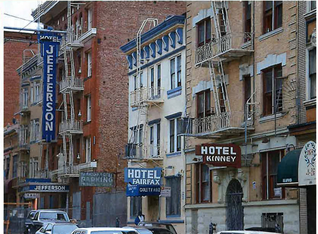
Jefferson Hotel, Built in 1906, 108 SRO units, Permanent Supportive Housing for Formerly Homeless Adults, Operator/Provider: Tenderloin Housing Clinic
